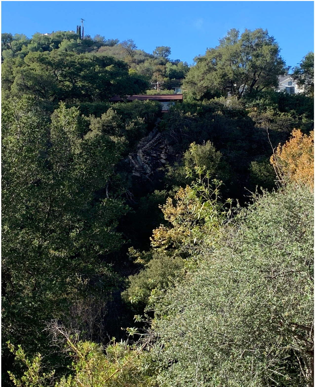
Figure 3.11. Private ladder on Mission Creek's right bank about 500 feet upstream from the debris dam. These access structures generate debris and promote accelerated weathering of the creek's canyon walls.
