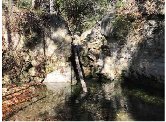
Figure 4.1.29: Potential impediment to fish passage at the remnants of an old dam constructed as part of the Santa Barbara Mission water supply system. The pool below is ~1.5 m deep and the dam creates a 2.5 m jump (right). Photos taken on February 4th, 2022 during drought base flow conditions.
