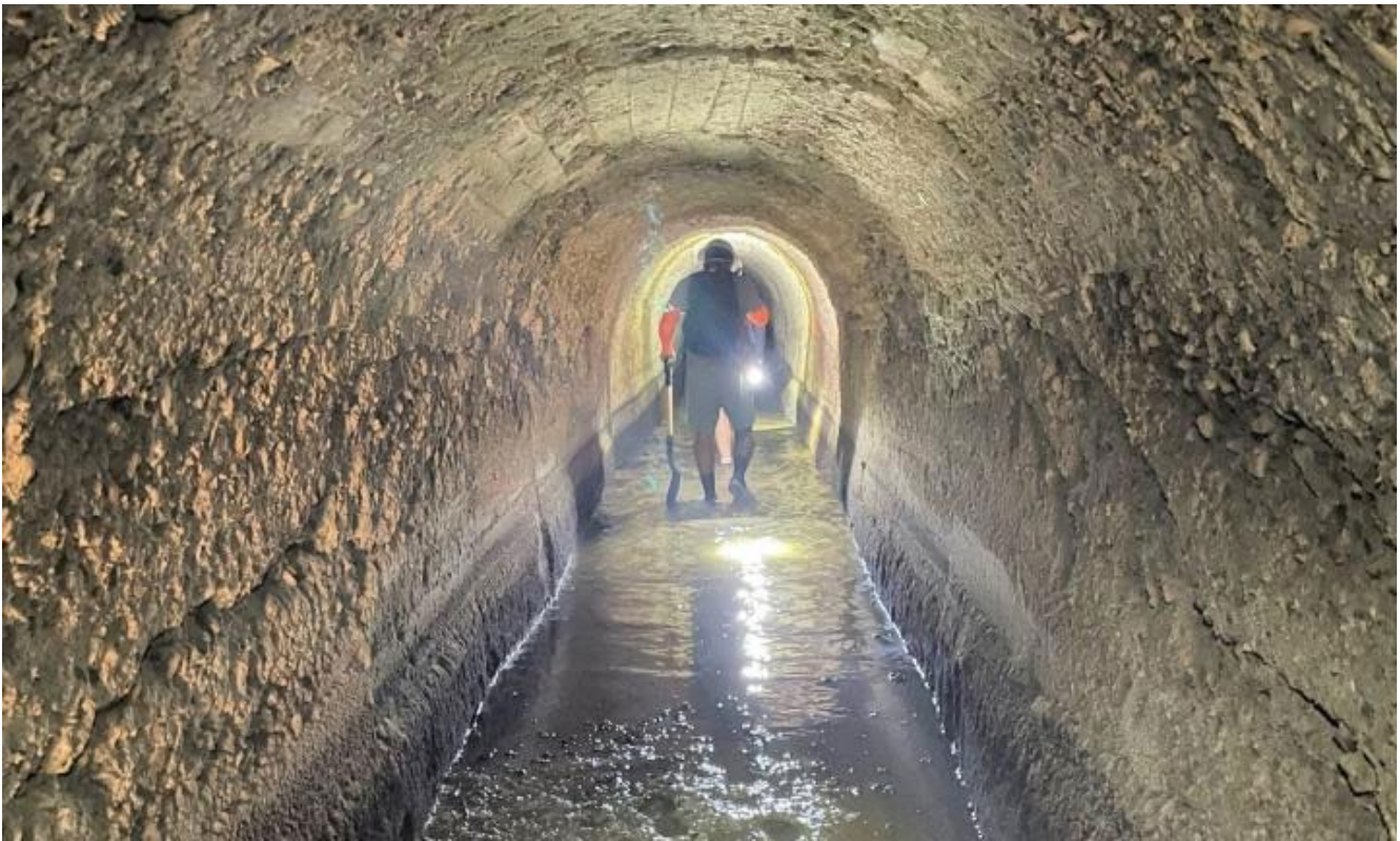
Figure 6.2. Photo of the interior of Mission Tunnel.
