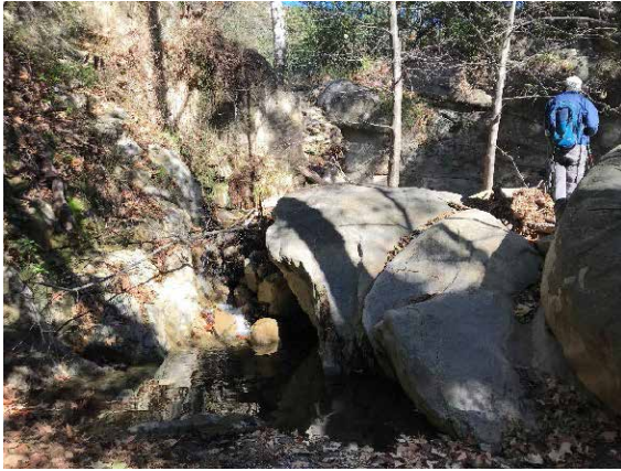
Figure 4.1.29: Potential impediment to fish passage at the remnants of an old dam constructed as part of the Santa Barbara Mission water supply system. The pool below is ~1.5 m deep and the dam creates a 2.5 m jump (right). Photos taken on February 4th, 2022 during drought base flow conditions.
