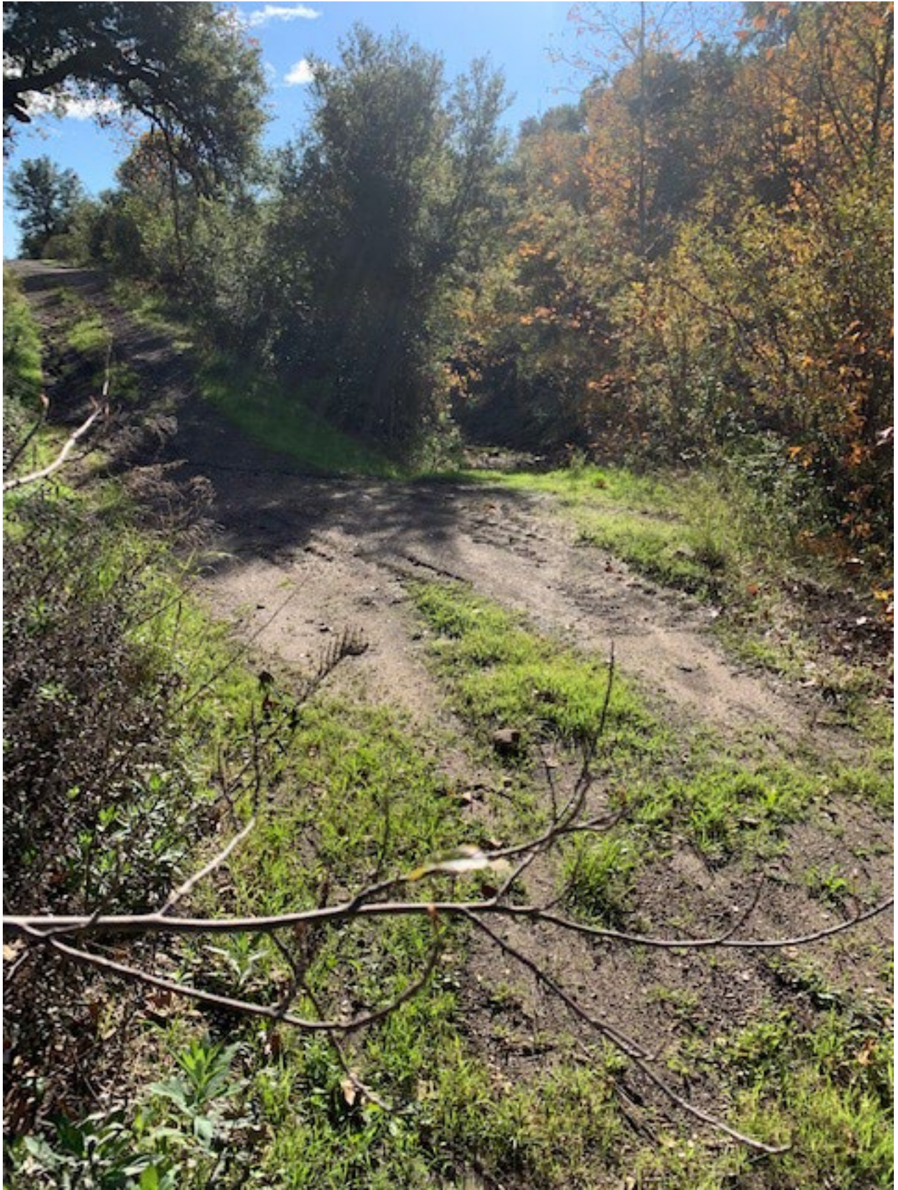
Figure 3.5. Access road to Mission Creek debris basin on the creek's left bank upstream from the basin.
