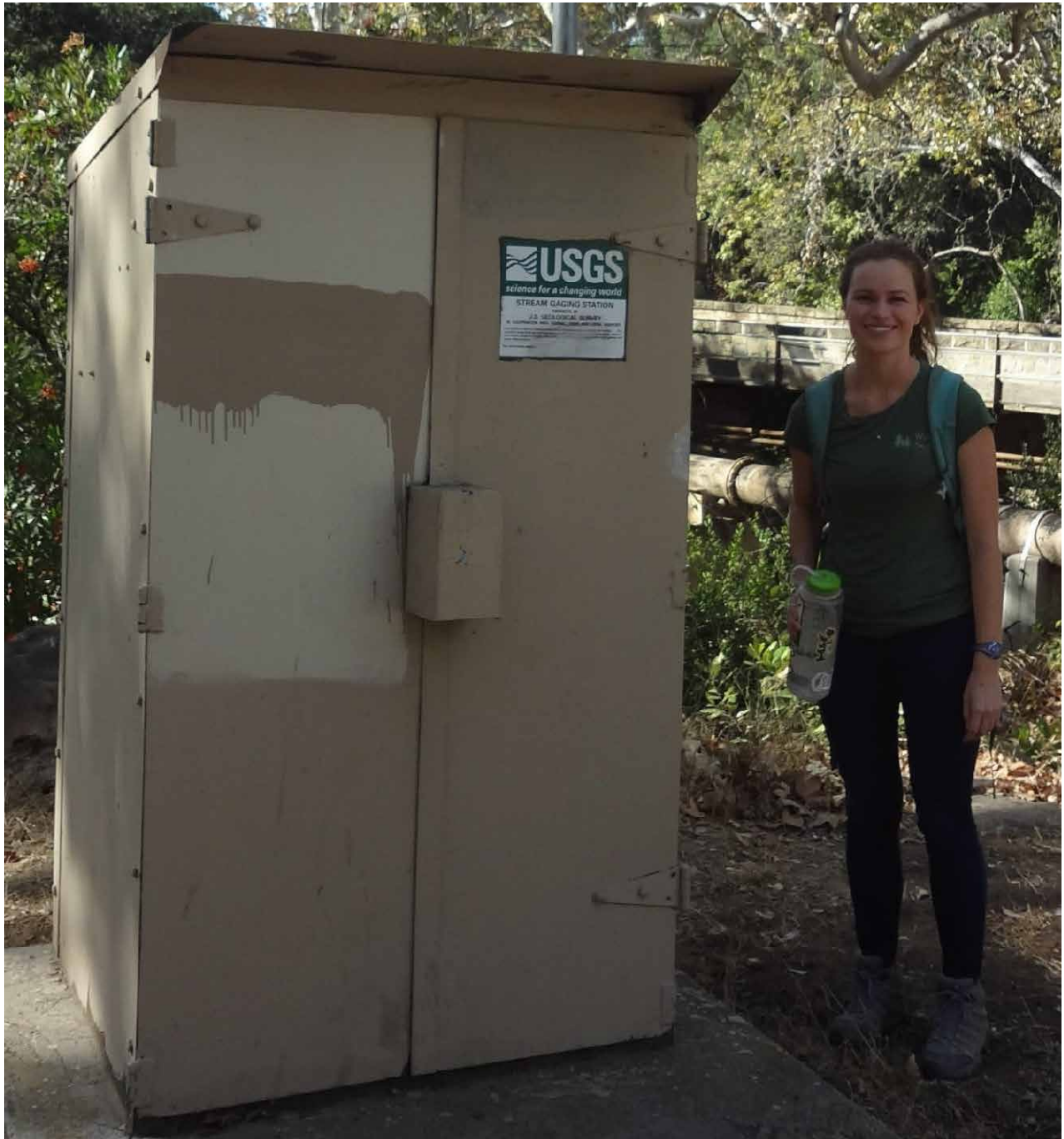
Figure 2.11. The control box for the USGS stream-gaging station # 11119745 at Rocky Nook Park. Paige Tripp poses for scale. The stone bridge on Mission Road over Mission Creek is seen in the background.
