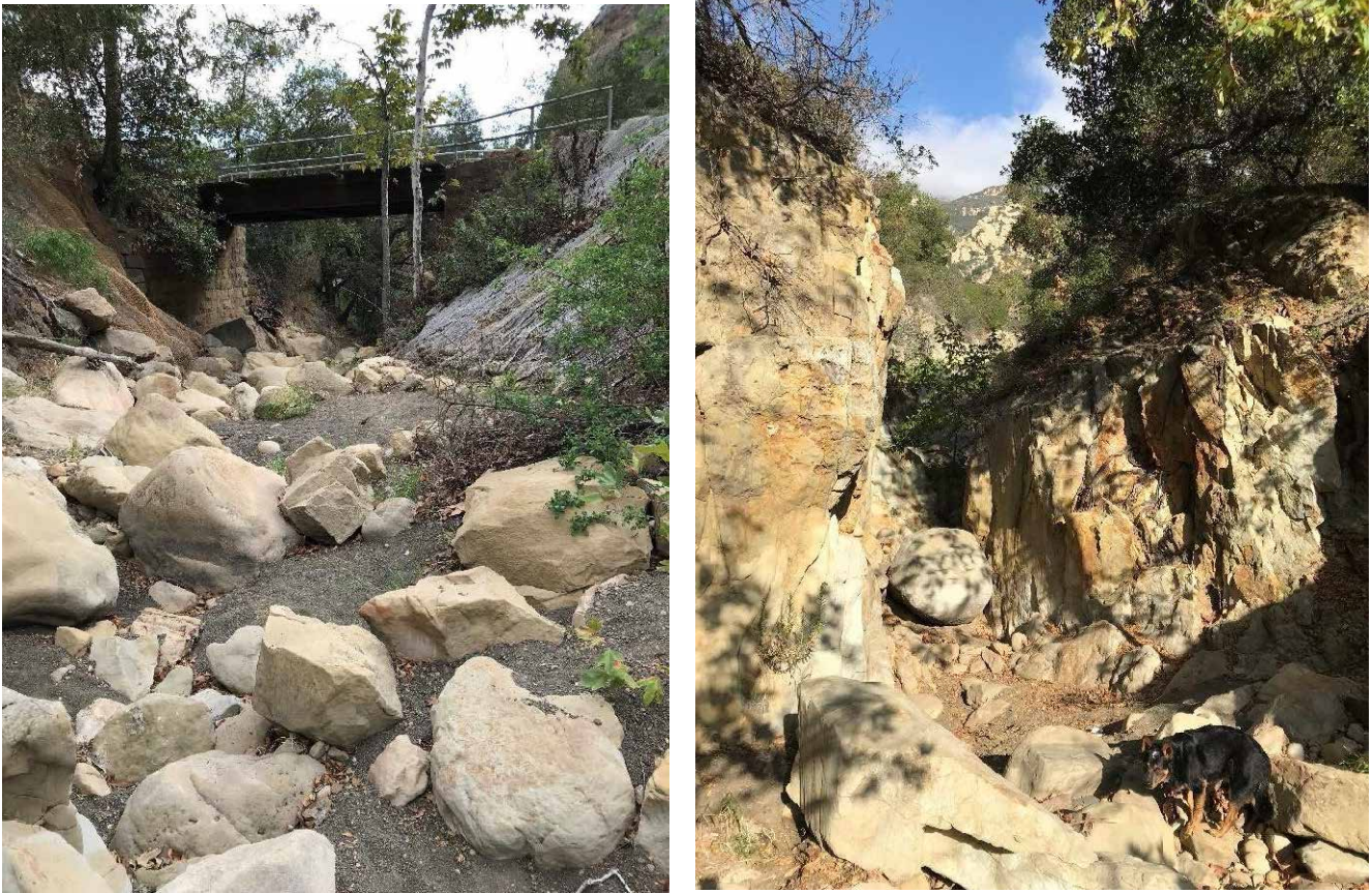
Figure 4.1.16. Small step pools, gravel deposits, and bedrock outcrops upstream of the Tunnel Rd. bridge (left). Narrow channel and plunge pool created by fractured bedrock (right). Photos taken on December 8, 2021 during base flow conditions.
