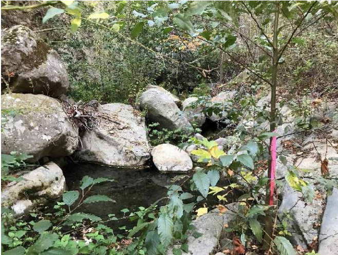
Deep pool downstream of the Tunnel Rd. bridge. Photo taken on December 12 th , 2021, during base flow conditions.
