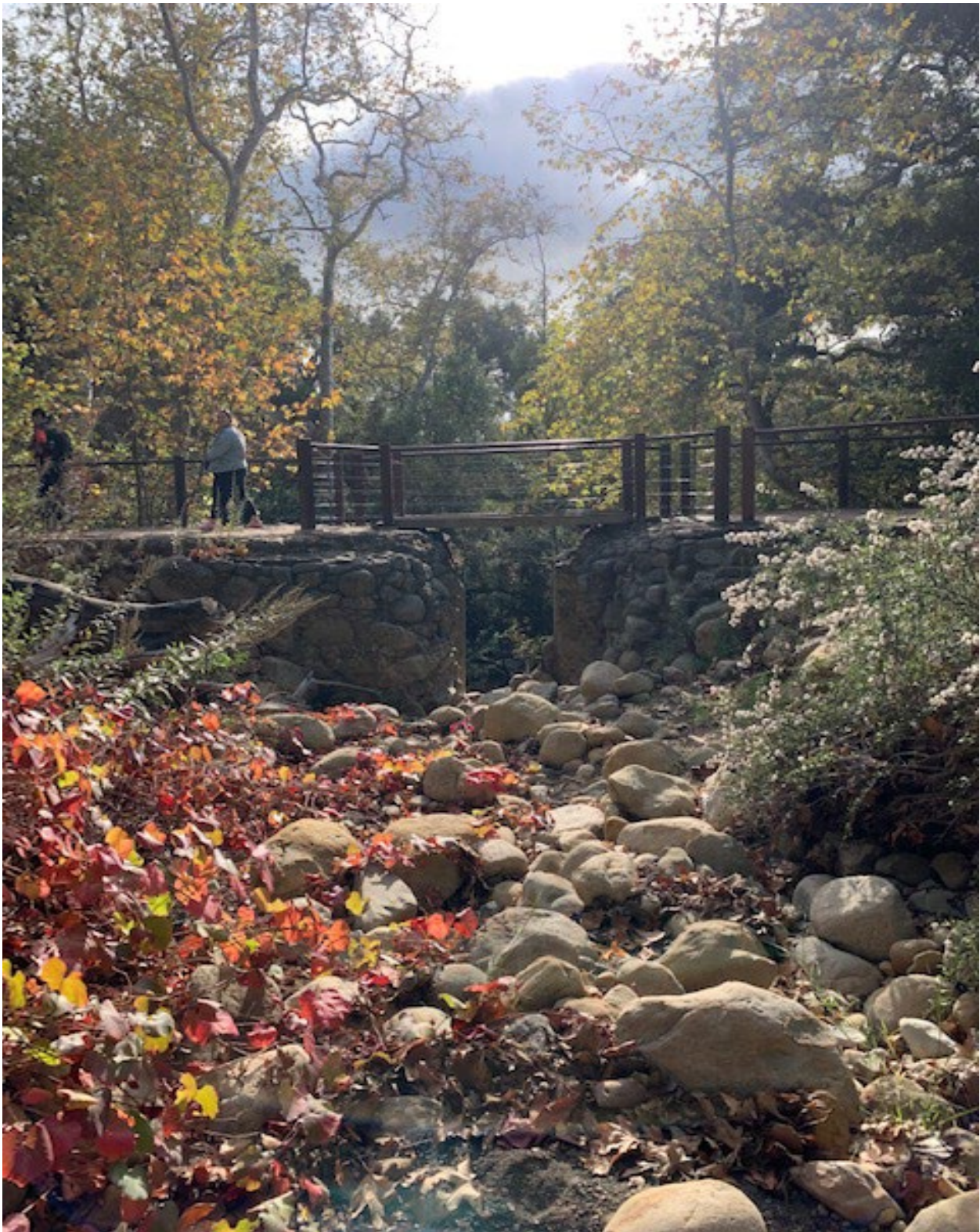
Figure 3.2. Photo of Mission Dam looking downstream. Large-size bedload is seen upstream Mission Dam.
