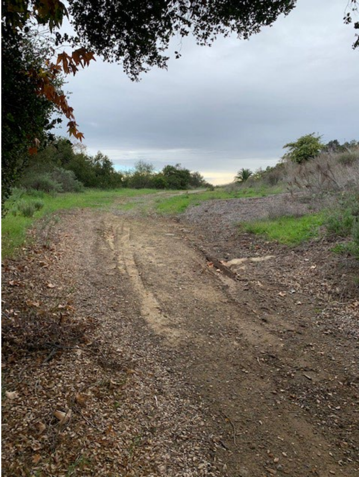
Figure 3.22. Access road and fill area for sediment dredged from the Rattlesnake Creek debris dam and basin. Photograph looking south.
