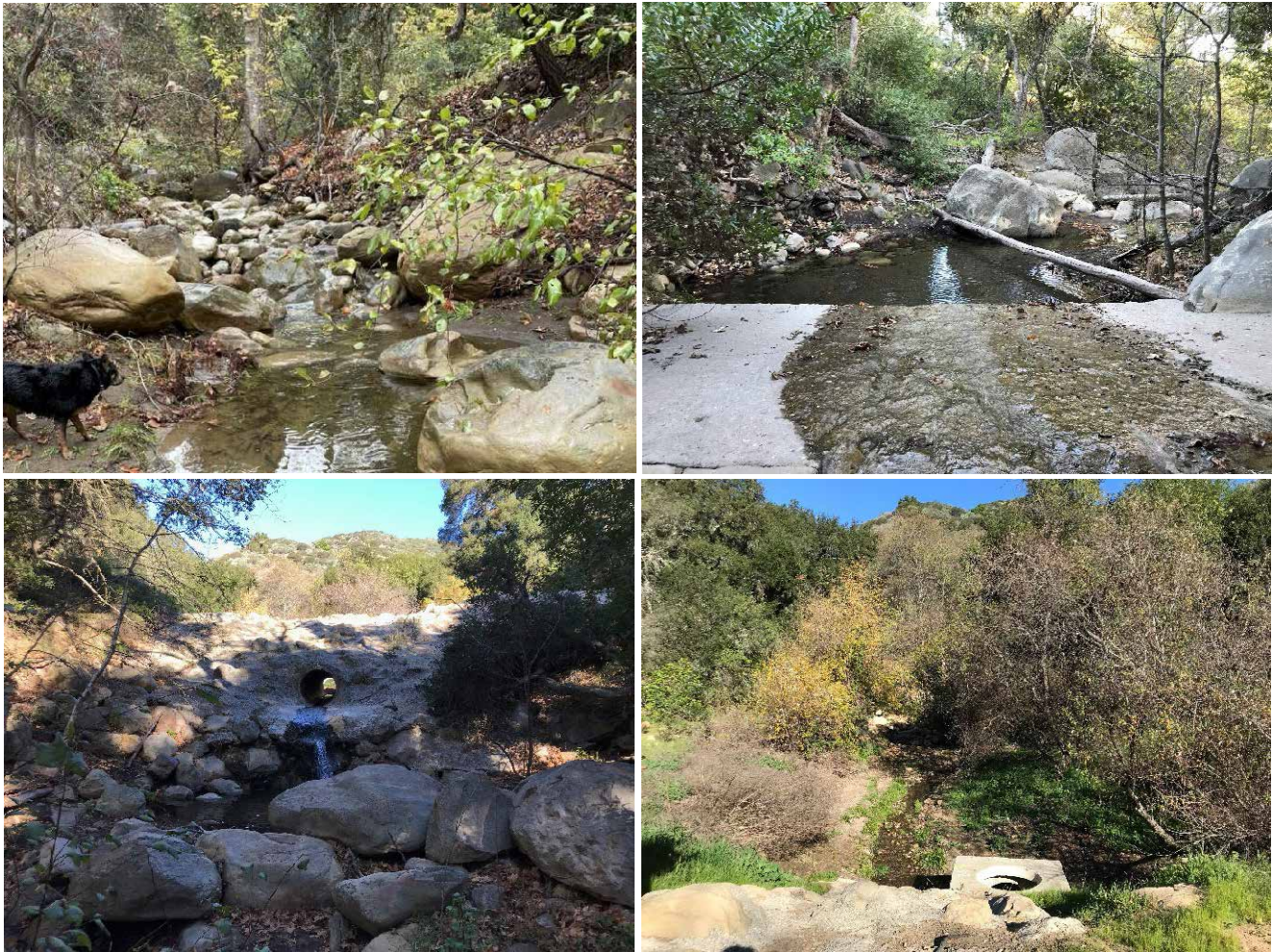
Figure 4.1.26. The relative proportion of large boulders (> 1-2 m in diameter) within the channel increases upstream through the Skofield Park reach (top left). View looking downstream of the concrete invert at the Las Canoas Rd. bridge (top right). A plunge pool formed by the concrete culvert creates a ~2m high jump and flow within the culvert that may impede or prevent fish passage/migration upstream during high stream flows. At the downstream end of the flood control debris basin (bottom left), a plunge pool formed below the culvert through the concrete dam creates a ~2 m high jump and the top of the debris dam is ~6 m above the water surface. Sediment deposition upstream of the dam inhibits pool development (lower right). Photos taken during low flow conditions on February 4th, 2022.
